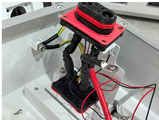
No.4.5-10 Inspection after test
