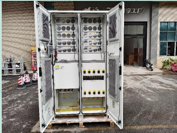
Fig 13 Internal inspection after test
