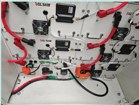
Fig 33 Internal inspection after test
