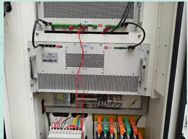
Fig 16 Internal inspection after test
