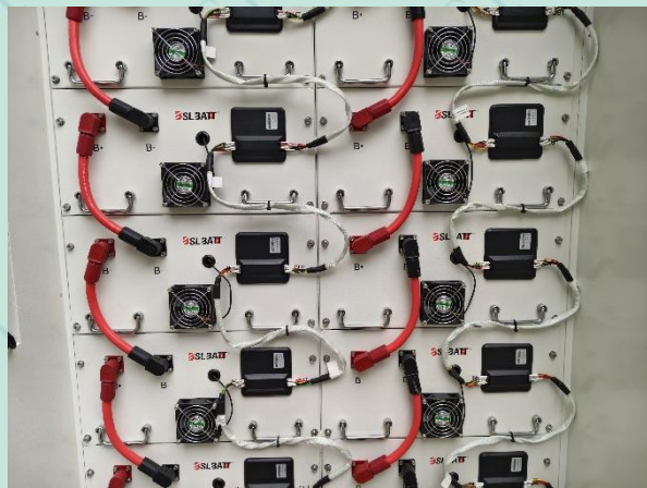
Fig 13 Internal inspection after test
