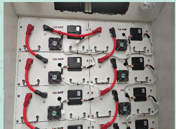
Fig 34 Internal inspection after test
