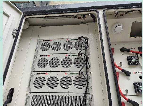
Fig 14 Internal inspection after test
