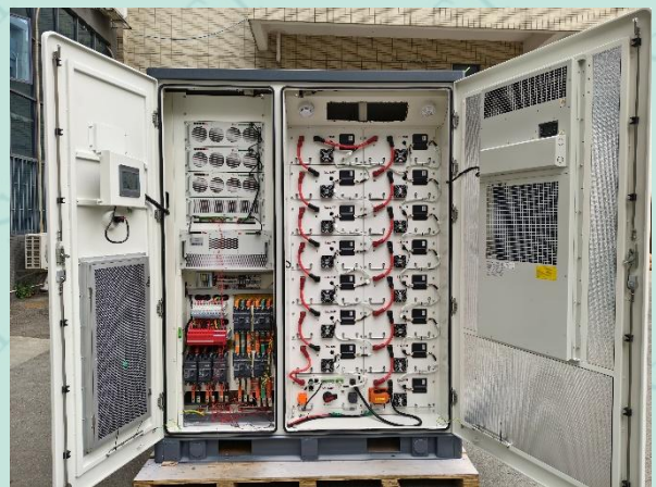
Fig 12 Internal inspection after test
