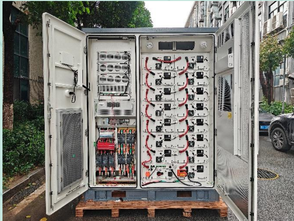
Fig 31 Internal inspection after test
