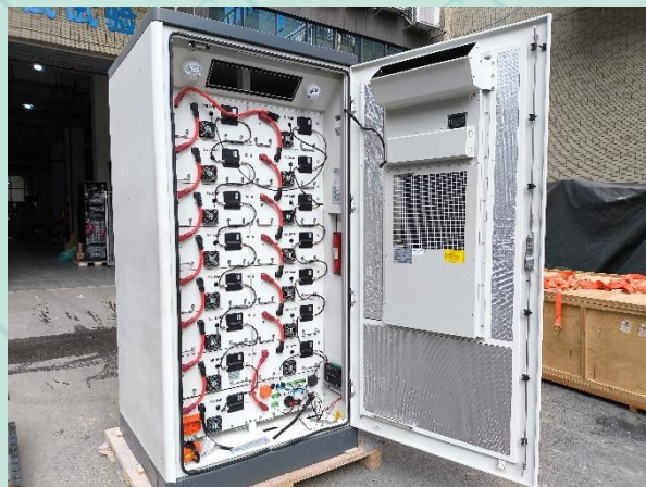
Fig 13 Internal inspection after test
