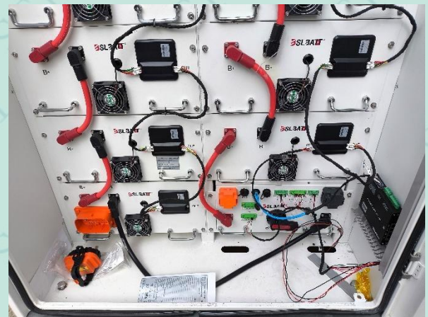
Fig 14 Internal inspection after test
