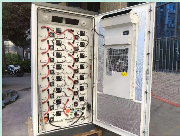
Fig 25 Internal inspection after test
