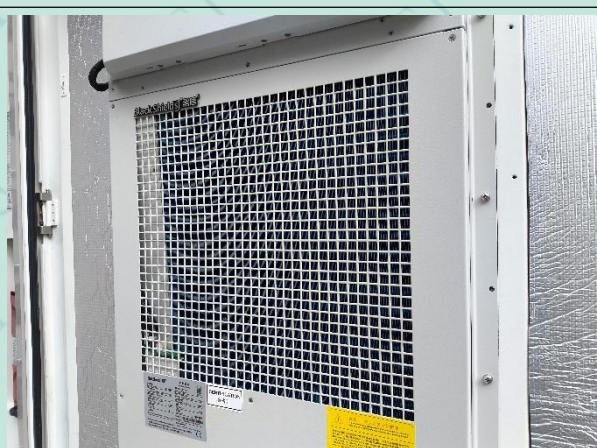
Fig 12 Internal inspection after test
