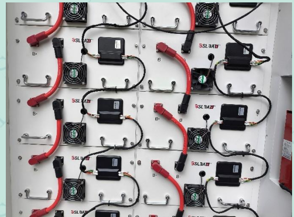
Fig 16 Internal inspection after test
