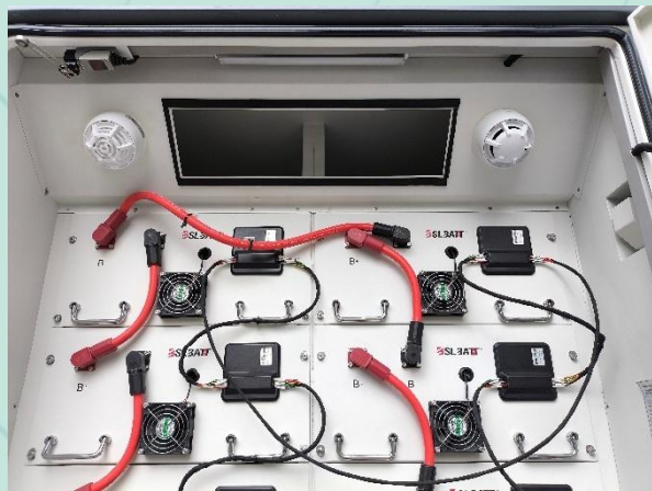
Fig 15 Internal inspection after test
