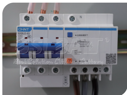
5 充电机总开关拨至ON档 The main switch of the charger is switched to ON.
