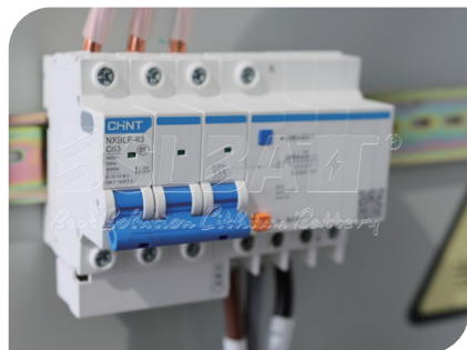
1 充电机总开关拨到OFF档 The main switch of the charger is switched to OFF.
