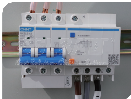
2 连接上充电机上AC端线束 Connect the AC terminal harness on the charger.
