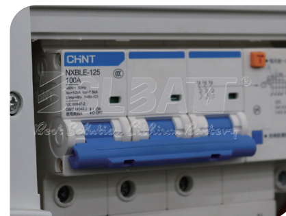
5 续第三步, 关闭充电机总开关 Continuing from step 3, switch off the main charger switch.
