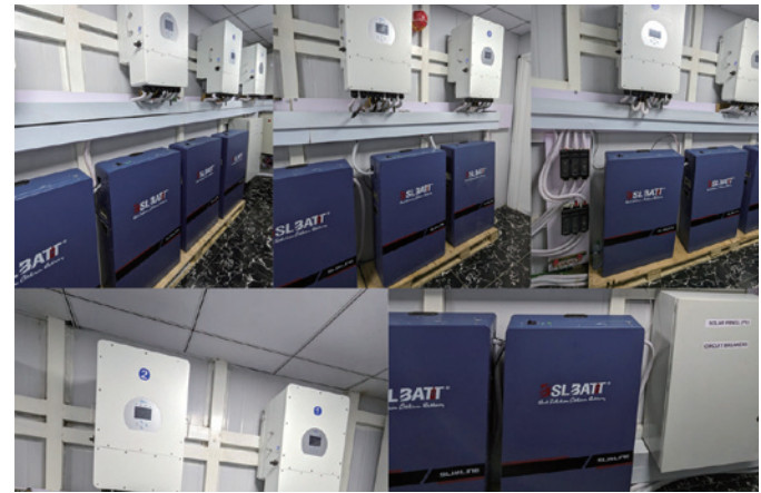
96kW Deye Inverter / 10*B-LFP48-300PW 153kWh / 120kWp Panel
