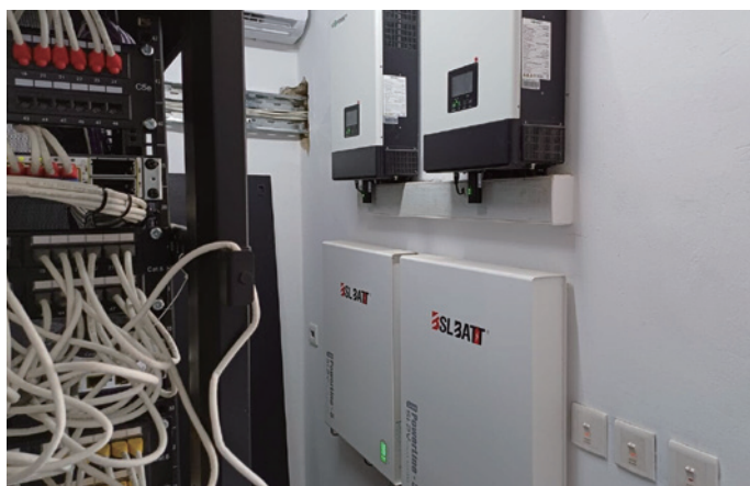
2* PowerLine-5 10kWh
