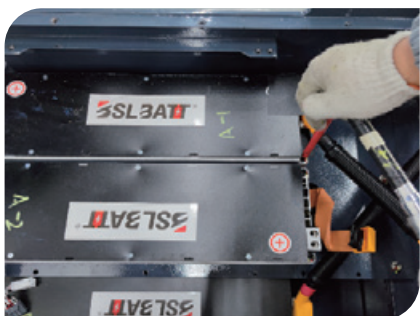
5 用13N*m紧固模组上的螺丝和螺杆 Tighten the screws and bolts on the module with 13N*m
