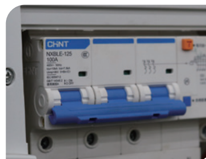
5 续第三步，关闭充电机总开关 Continue to the third step, turn off the main switch of the charger
