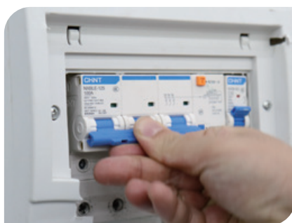
4 AC端总开关拨至ON档 Turn the AC terminal main switch to ON position
