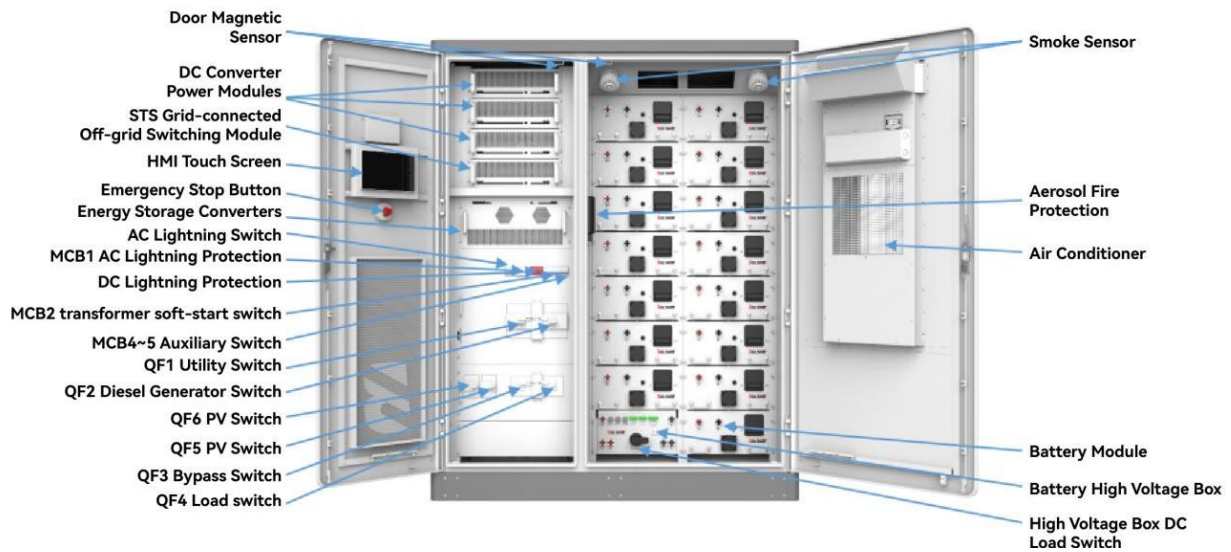
Figure 4.1 Location diagram of power distribution switch
