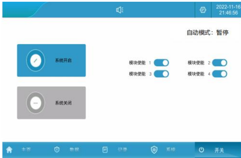
Figure 5.17 Automatic control operation mode is turned on
